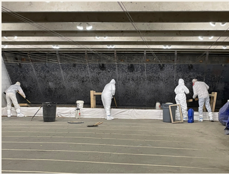
Leveling The Lead Receiver Pit
